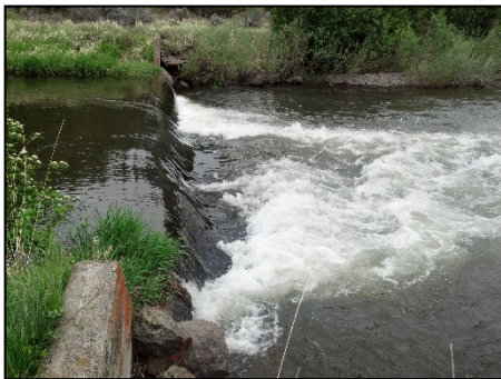
Page Springs Weir – Donner & Blitzen River
