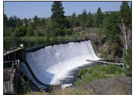
North Unit Dam – Deschutes River
